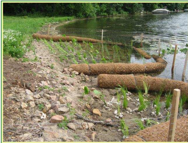
Biologs are an effective tool in the fight against shoreline erosion and protect the new plantings until they are established.
